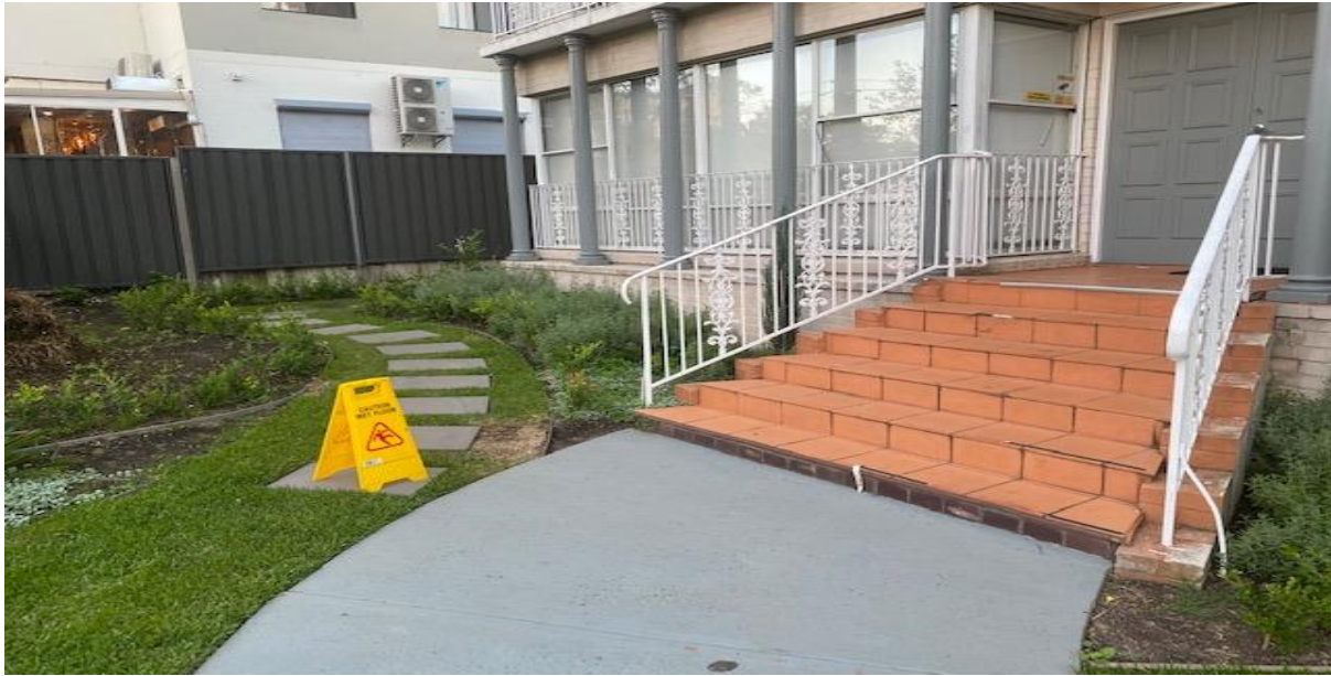
Another photo showing the principal pedestrian entrance requiring a chair lift. Accessible Entrance signage will also be required for this area.
