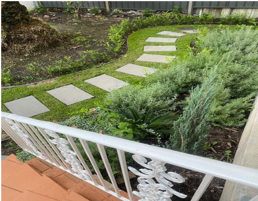
Photo showing none complying grassed access pathway to be made compliant with AS1428.1.
